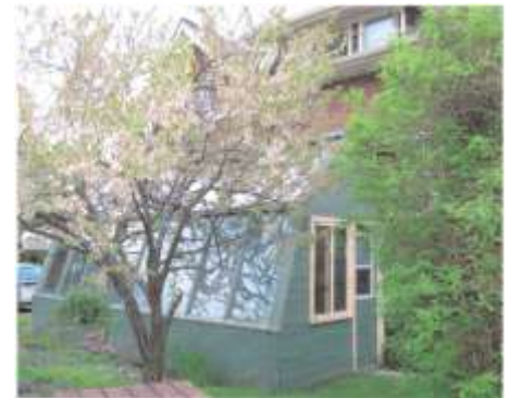
Susan and Maurice Grinstead have been heating their home with a passive solar greenhouse for 30 years. Photo submitted by Susan Grinstead.
